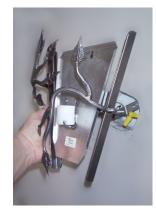
Wirec connected to wall box Fixture bracket attached to wall box
